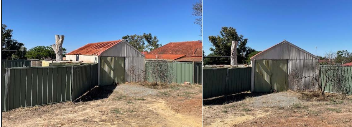
Figure 11.2.5 – View from Irwin Street of existing shed to be demolished for proposed shed
