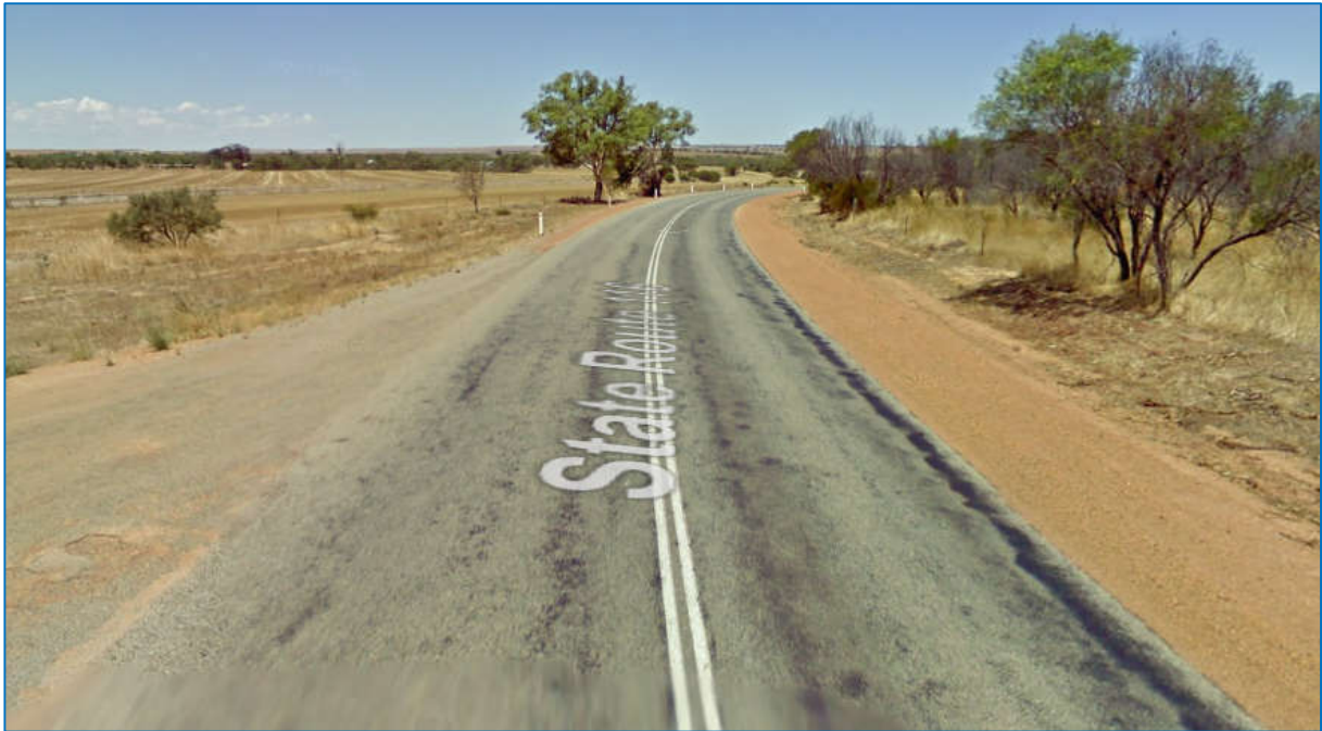
Figure 10: Midlands Road Looking East
