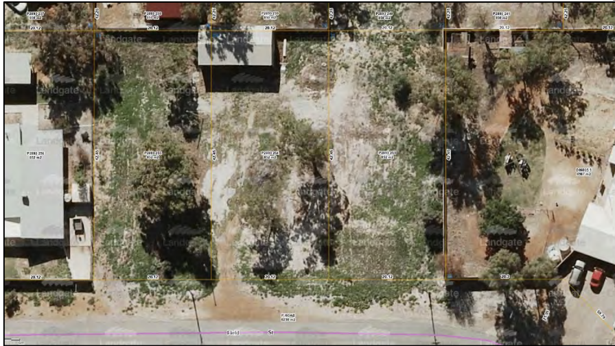
Figure 11.4(b) – Aerial Photo of 21 (Lots 253, 254 & 255) Field Street, Mingenew
