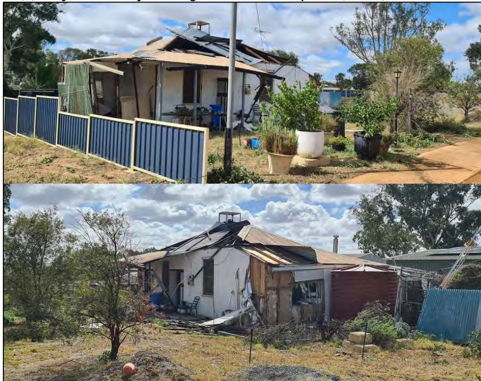
Figure 6.1(d) – Cyclone Seroja damage to residence upon 6 (Lot 16) Bride Street, Mingenew
