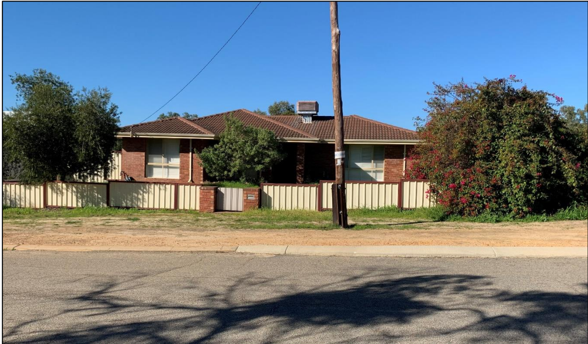
Figure 11.1(c) – View of Lot 137 looking east from Enanty Street
