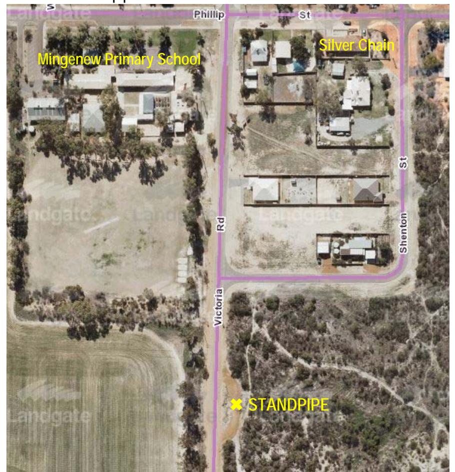
Commercial Standpipe Location:
