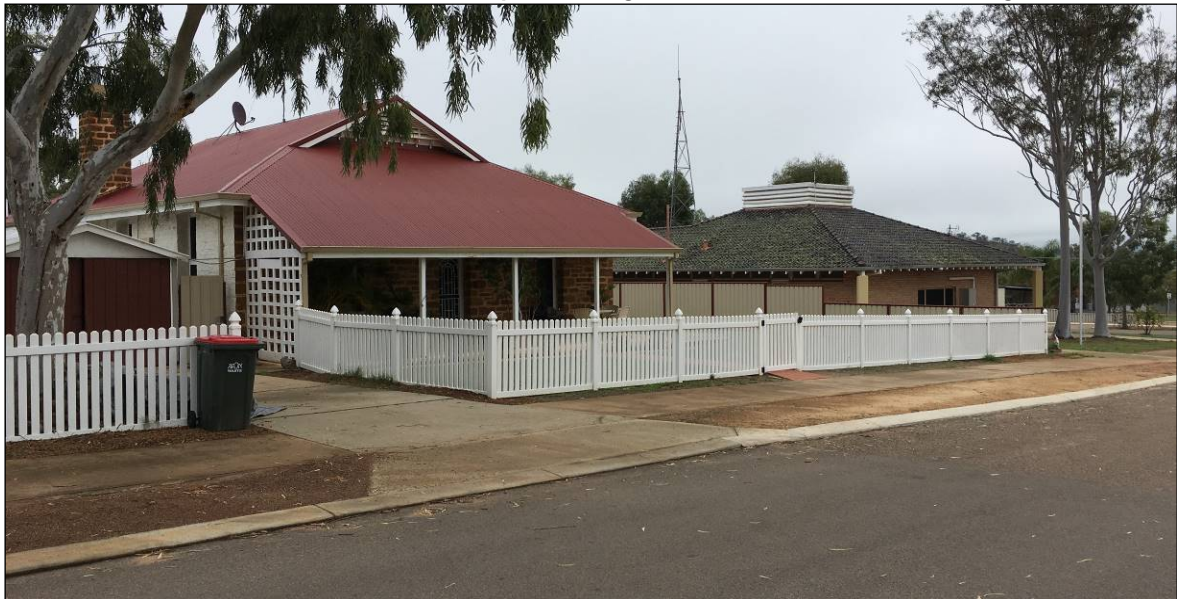
Figure 9.4.1(b) – View of former Mingenew Police Station upon Reserve 7422 looking north-west from William Street with subsequent Mingenew Police Station in background
