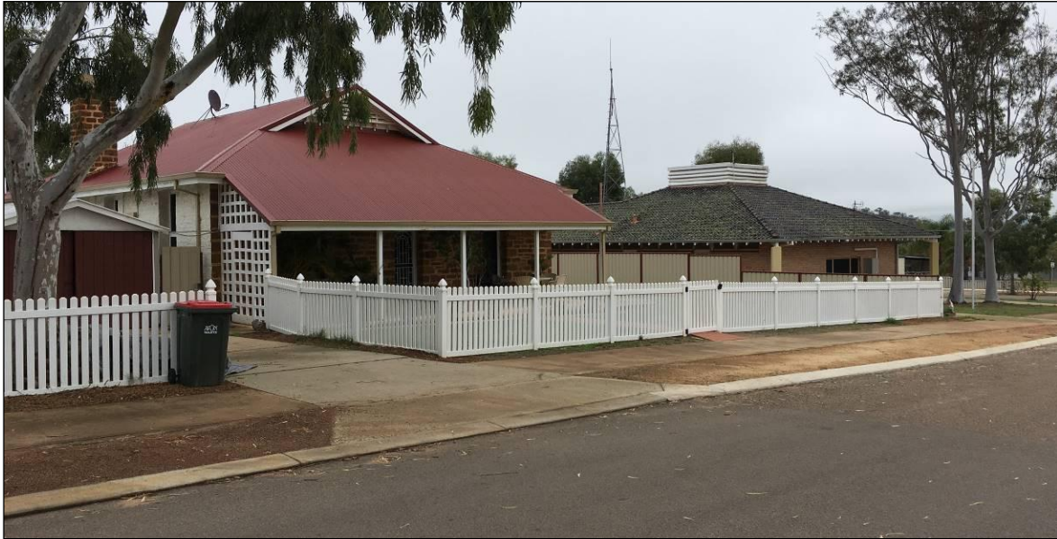
Figure 9.4.1(b) – View of former Mingenew Police Station upon Reserve 7422 looking north-west from William Street with subsequent Mingenew Police Station in background
