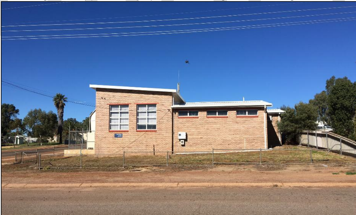
Figure 9.4.1(c) – View of proposed site looking south from King Street
