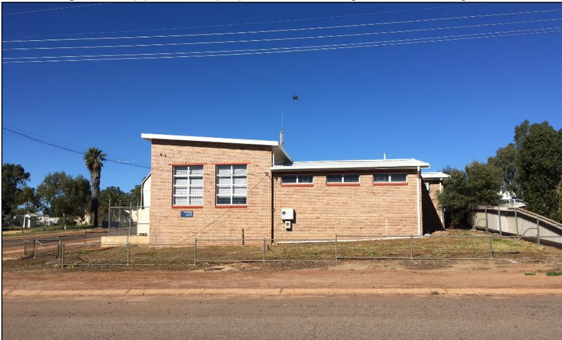
Figure 9.1.1(c) – View of proposed site looking south from King Street
