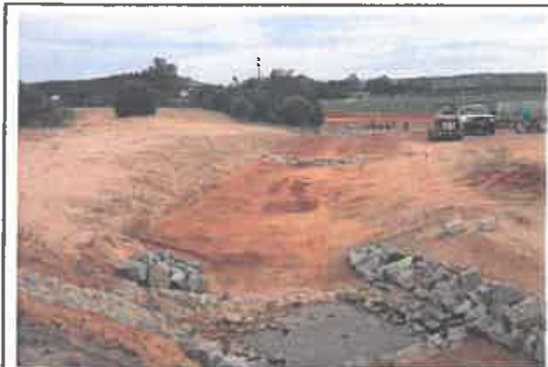
Further Photo of recently completed upgrade works at CBH Facility
