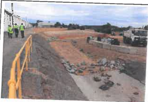
Recently Complete upgrade works within the CBH site
