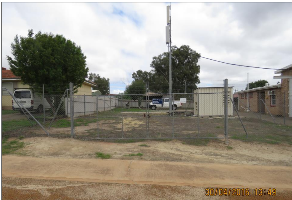
Figure 6: Existing site access gate off Shenton Street onto the subject property – Source : Visionstream
