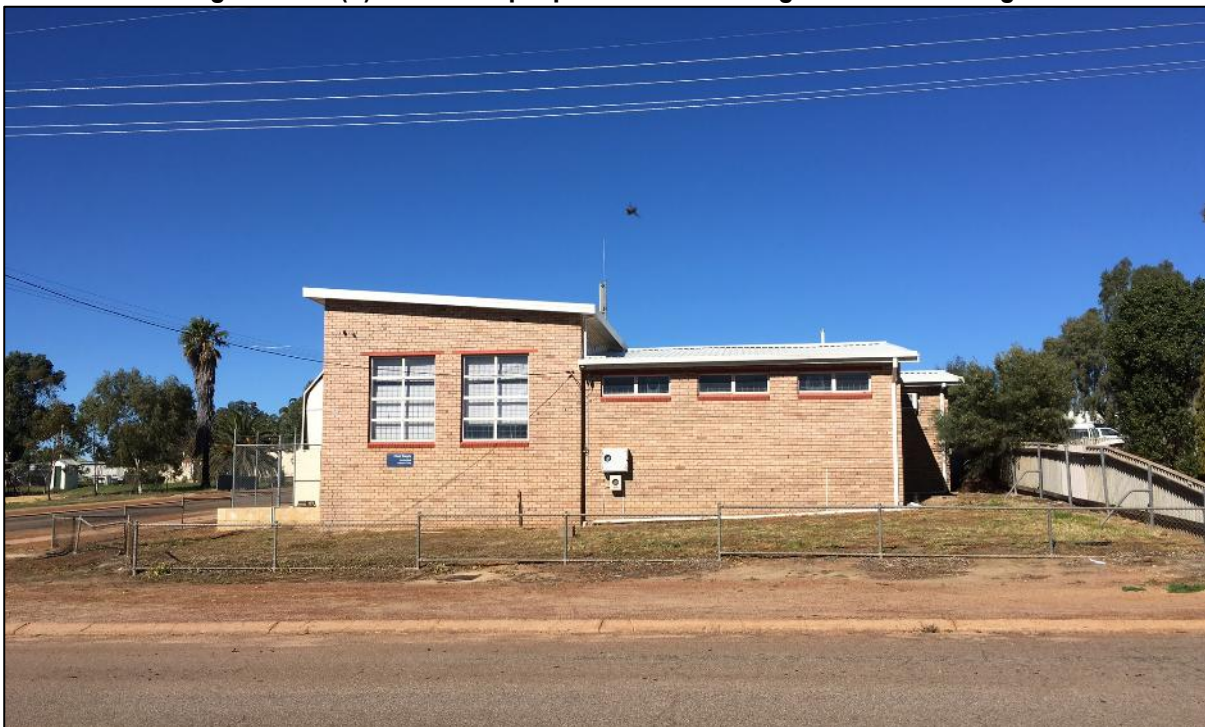
Figure 9.4.2(c) – View of proposed site looking south from King Street
