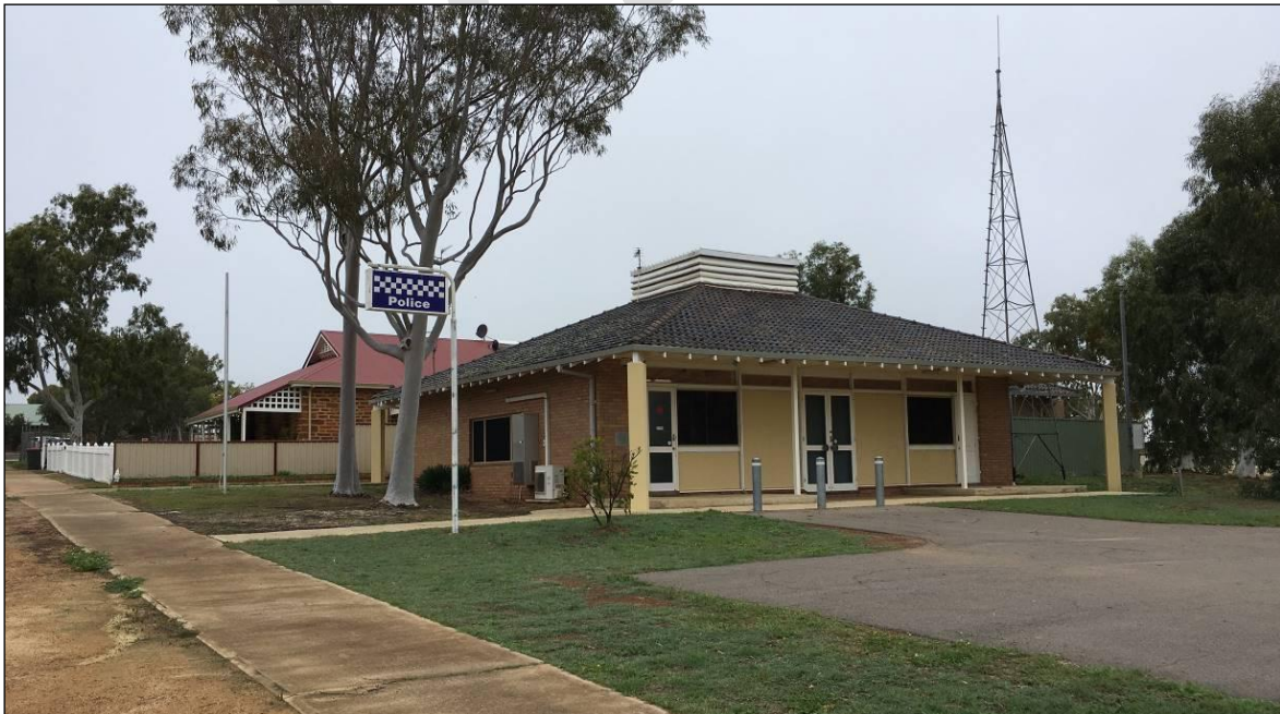
Figure 9.4.1(c) – View of Mingenew Police Station upon Reserve 24354 looking south-west from William Street with former Mingenew Police Station in background
