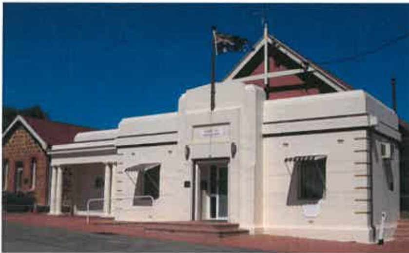
Plate 3 Shire of Administration Office
