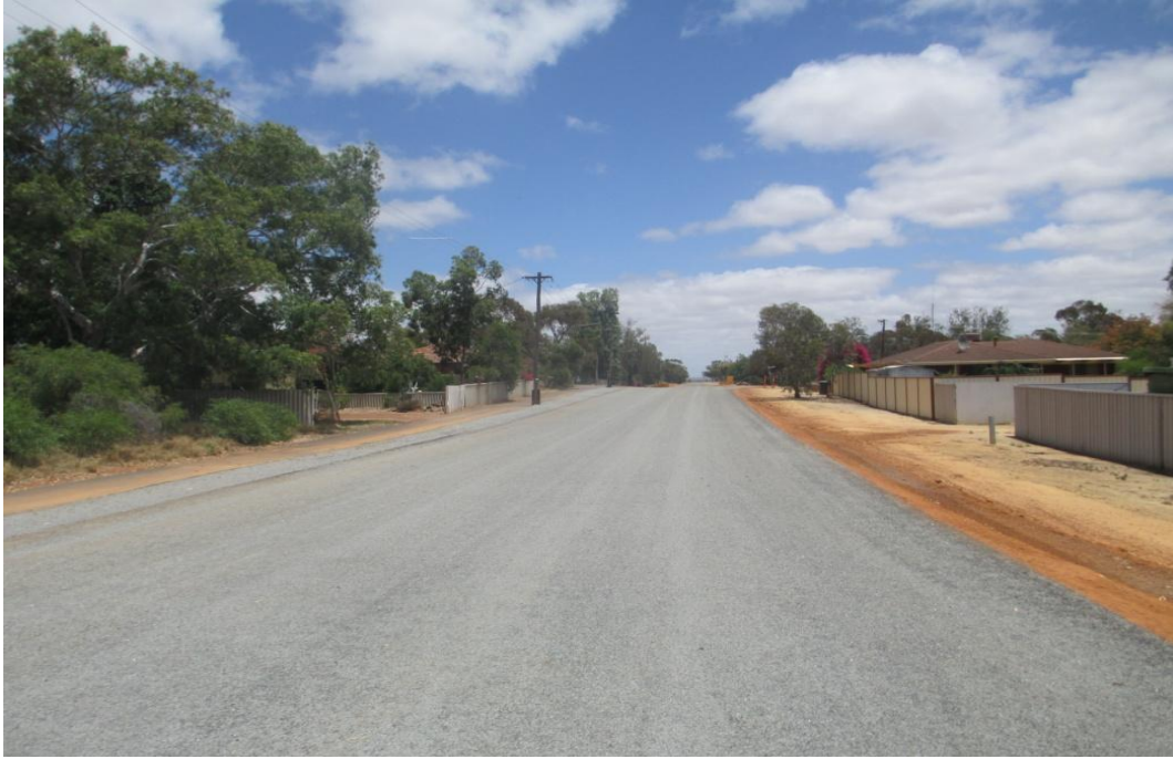
Moore Street Reconstruction
