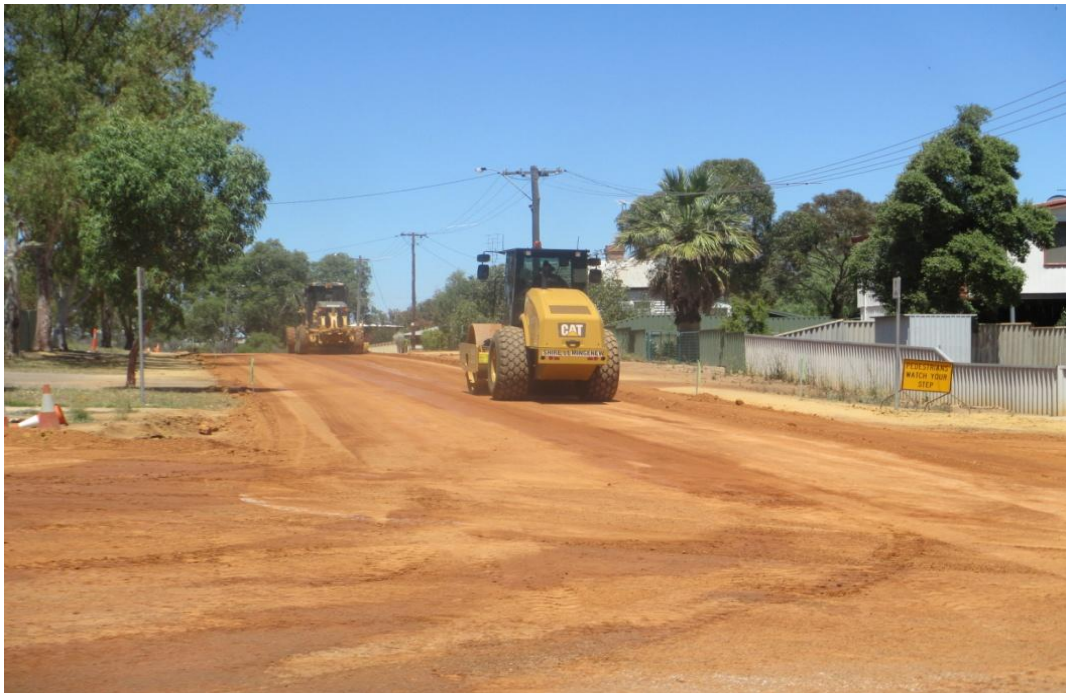
Moore Street Reconstruction
